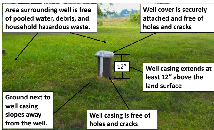
Figure 1: Photo of a properly constructed well.
